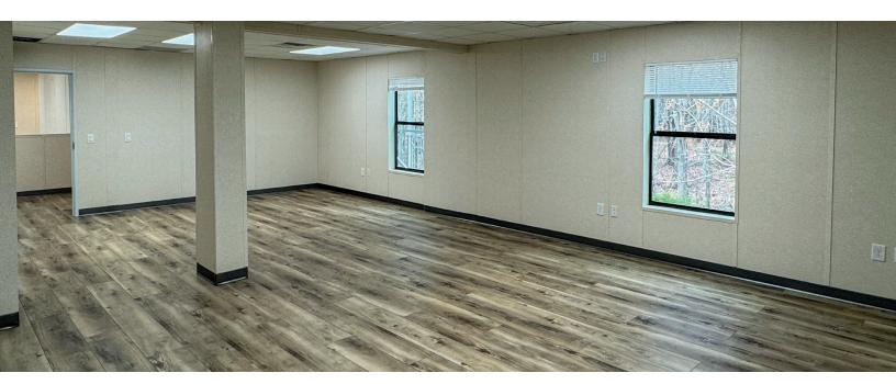
**Flooring:** Commercial-grade Roll Vinyl and Site-Finished LVT Flooring were selected for durability and ease of maintenance and installed throughout the facility to provide a robust and aesthetically pleasing environment.
